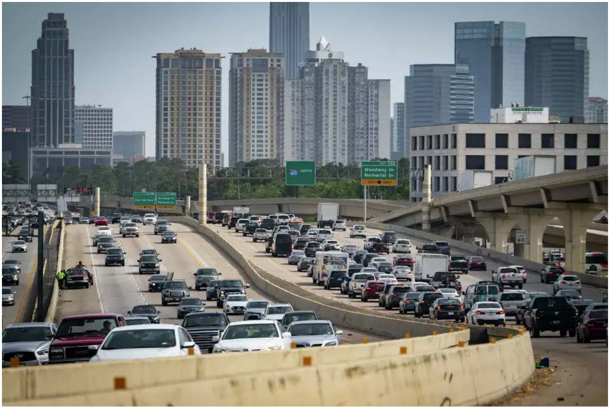
Figure B.8. Houston's I-610 Highway Loop
